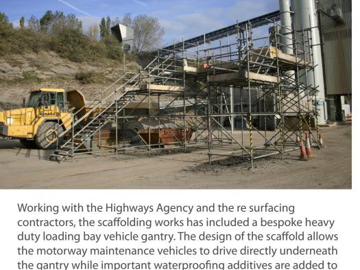
the hot bitumen. This enables the vehicles to drive straight on to the motorway thus reducing any unnecessary downtime and preventing any potential congestion on the motorway. The scaffolding gantry included: Pre-Planning Engineer Site Surveys Scaffold Designs & Calculations
